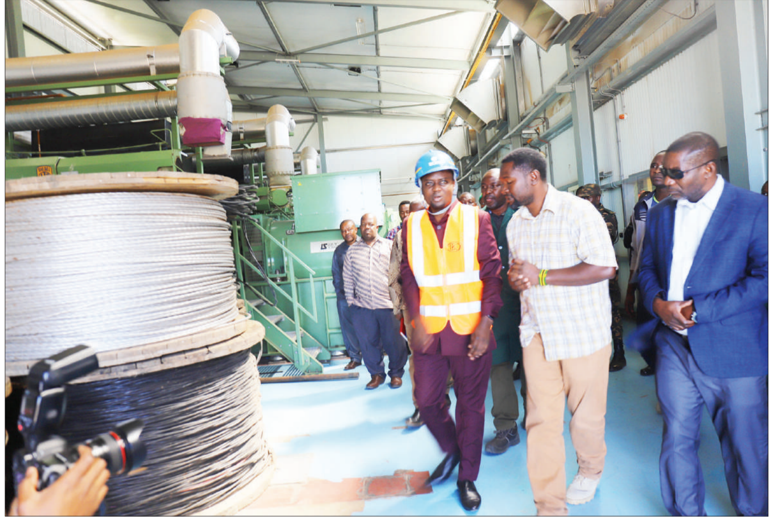
Arusha regional commissioner Mrisho Gambo (L, foreground) pictured at the weekend going around a power supply project supposed to serve Ngorongoro District but whose implementation is said to be experiencing an unnecessary delay. Photo: Correspondent Asraji Mvungi
