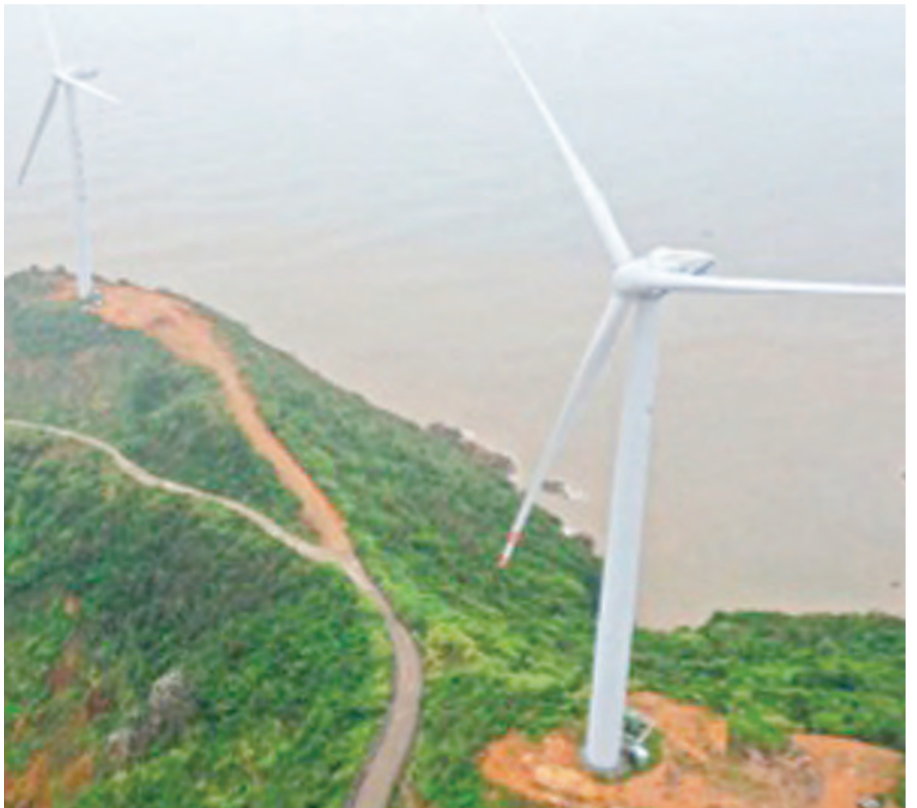
Photo taken on May 23, 2021 shows a wind farm in Yuhuan, east China's Zhejiang province. The wind farm has 25 wind turbines and an installed capacity of 49.5 megawatts. It is able to generate 120 million kWh of electricity on a yearly basis. Photo: People's Daily
