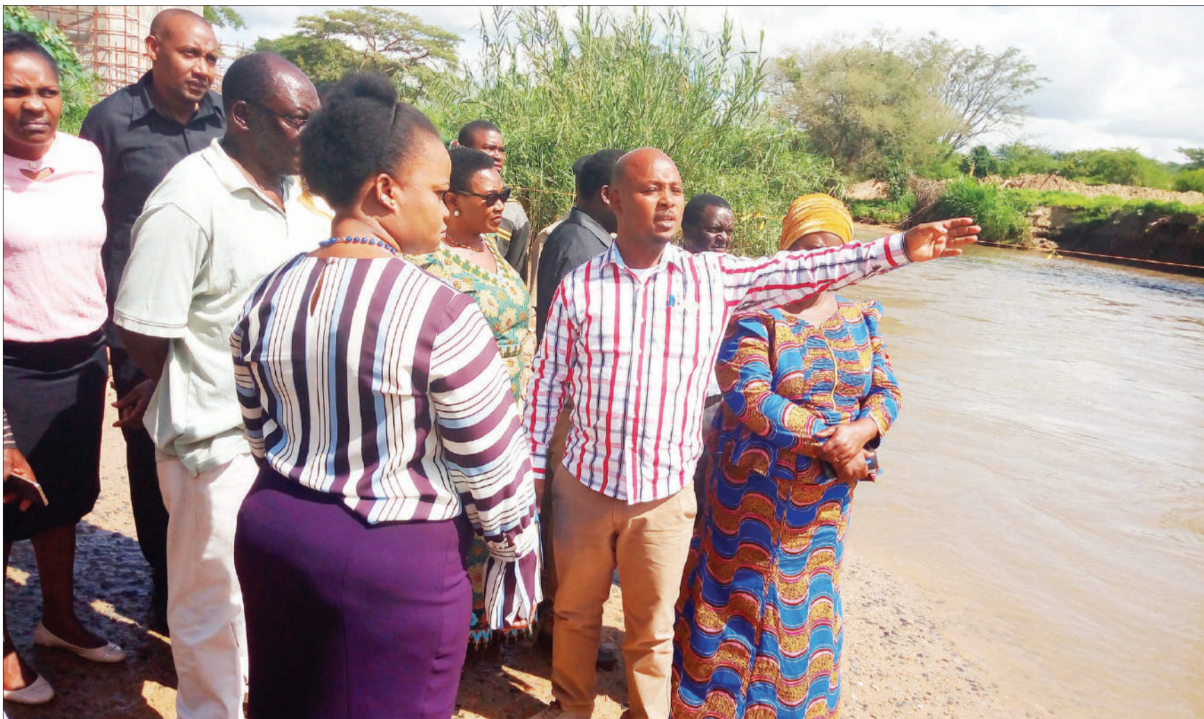
Tanzania National Roads Agency deputy regional manager in Mbeya Mageza Mwita (2nd R) briefs Chunya district commissioner Maryprisca Mahundi on the rehabilitation of Lupa bridge after it was closed for two weeks due to flooding yesterday. Photo: Correspondent Nebart Msokwa.
