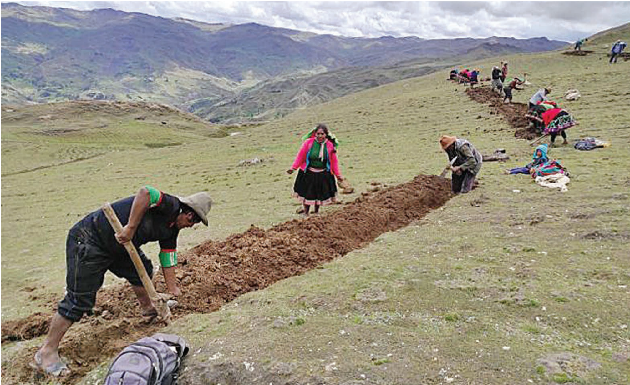
Women and men from the rural community of Sachac, at more than 3500 meters above sea level, build a kilometer-long infiltration ditch to capture rainwater and use it to irrigate crops in Cuzco, in Peru’s Andes highlands. CREDIT: Janet Nina/IPS
