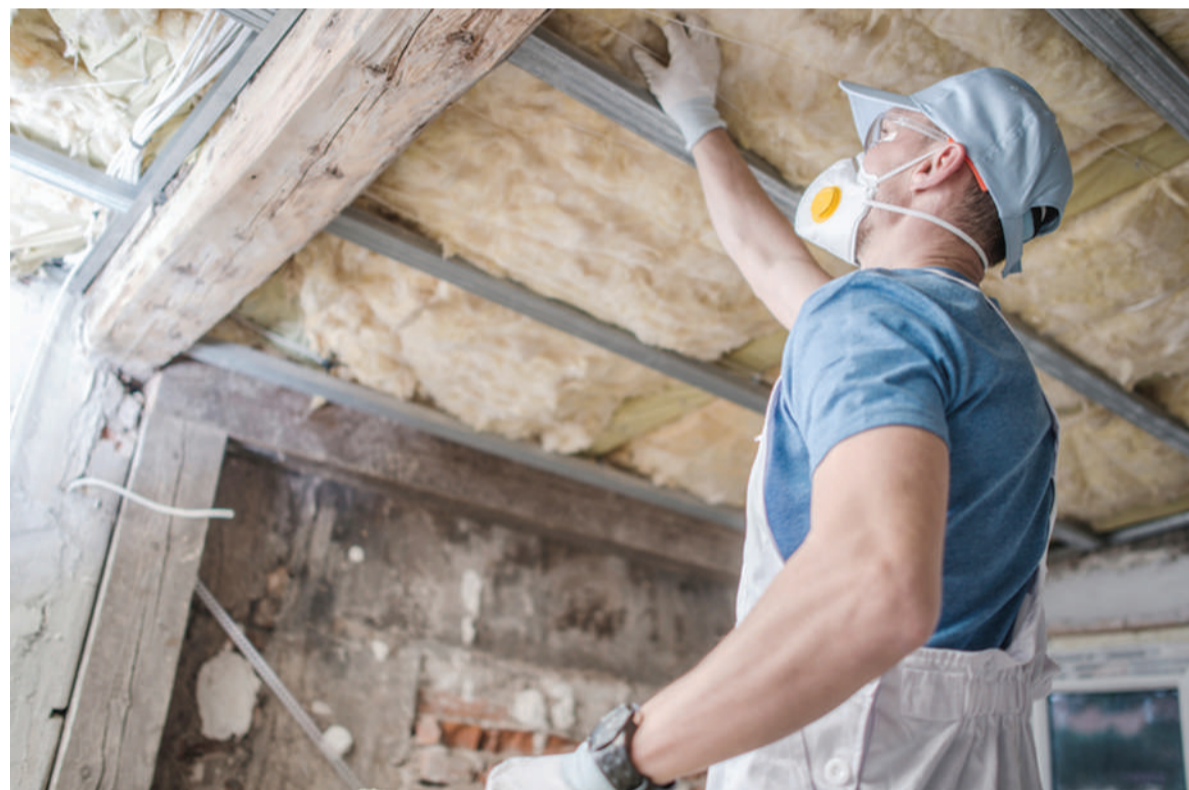
A man doing insulation installation
