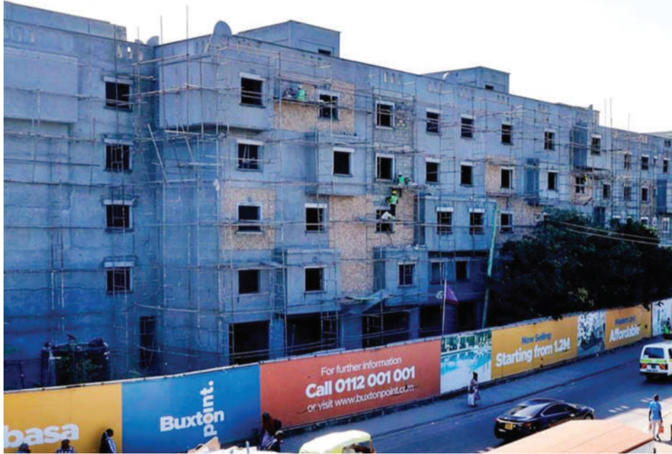
The ongoing construction of affordable housing at Buxton
