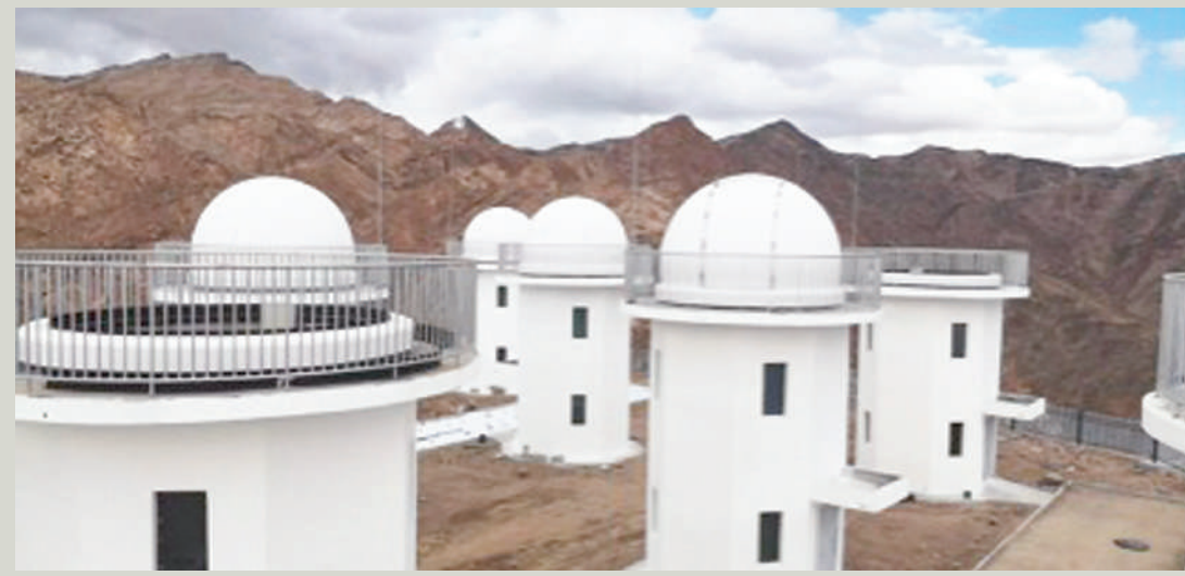
Photo shows a multi-application survey telescope array, or MASTA, deployed at a 3,800-meter-high platform of an astronomical observatory under construction in Lenghu, Mangya city, Haixi Mongol and Tibetan autonomous prefecture, northwest China's Qinghai Province. File photo
