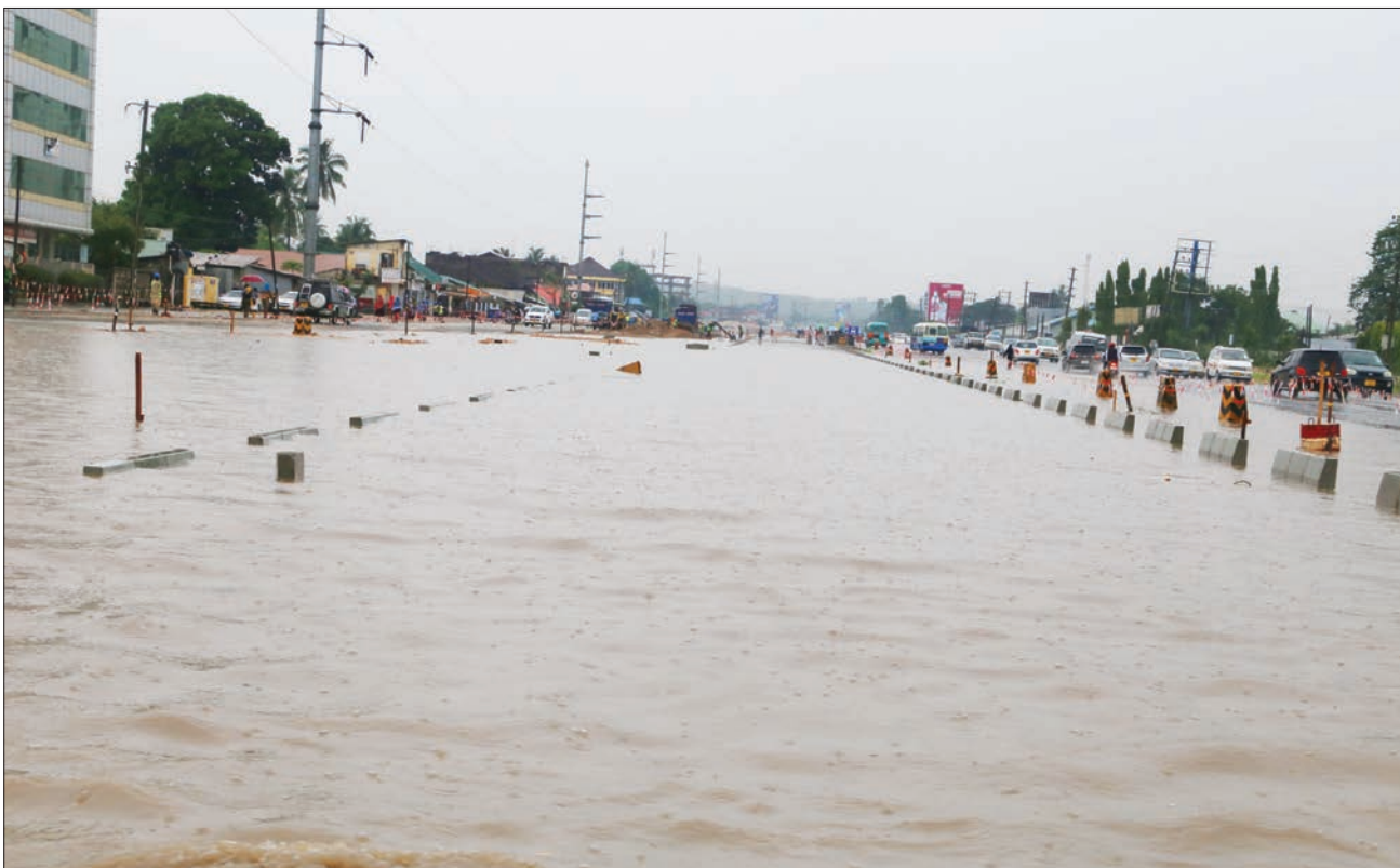
Even this stretch of Bagamoyo Road which is undergoing expansion was not spared by floodwaters.
