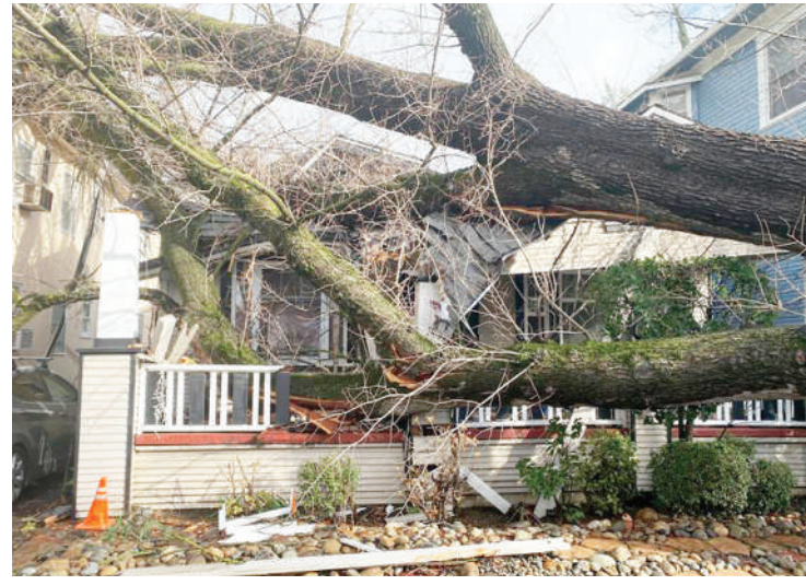
A tree collapsed and ripped up the sidewalk damaging a home in Sacramento, California on Sunday. AP
