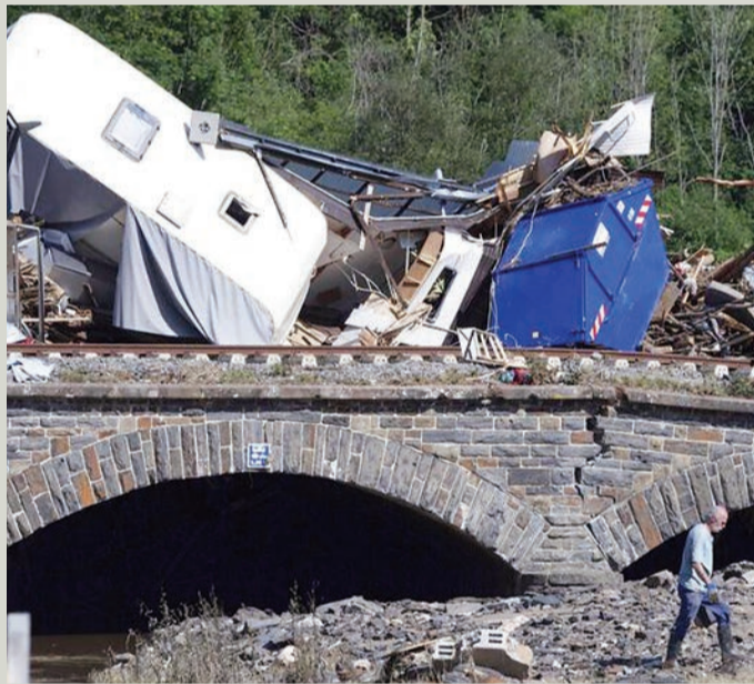
Caravans, cars and mobile homes that were swept away by the flood wave hang together on a bridge over the River Ahr, in Altenahr, western Germany on Sunday. AP
