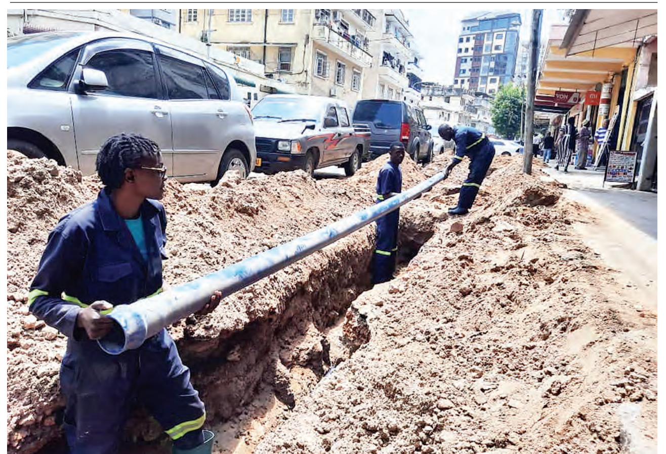
Dar es Salaam Water and Sanitation Authority (Dawasa) technicians replace a damaged water pipe along Jamhuri Street in Dar es Salaam at the weekend, chiefly with a view to improving water supply to residents of downtown Mosque, Libya, Mshihiri, Kitumbini, Aggrey and Moscow streets. Photo: Correspondent Joseph Mwendapole
