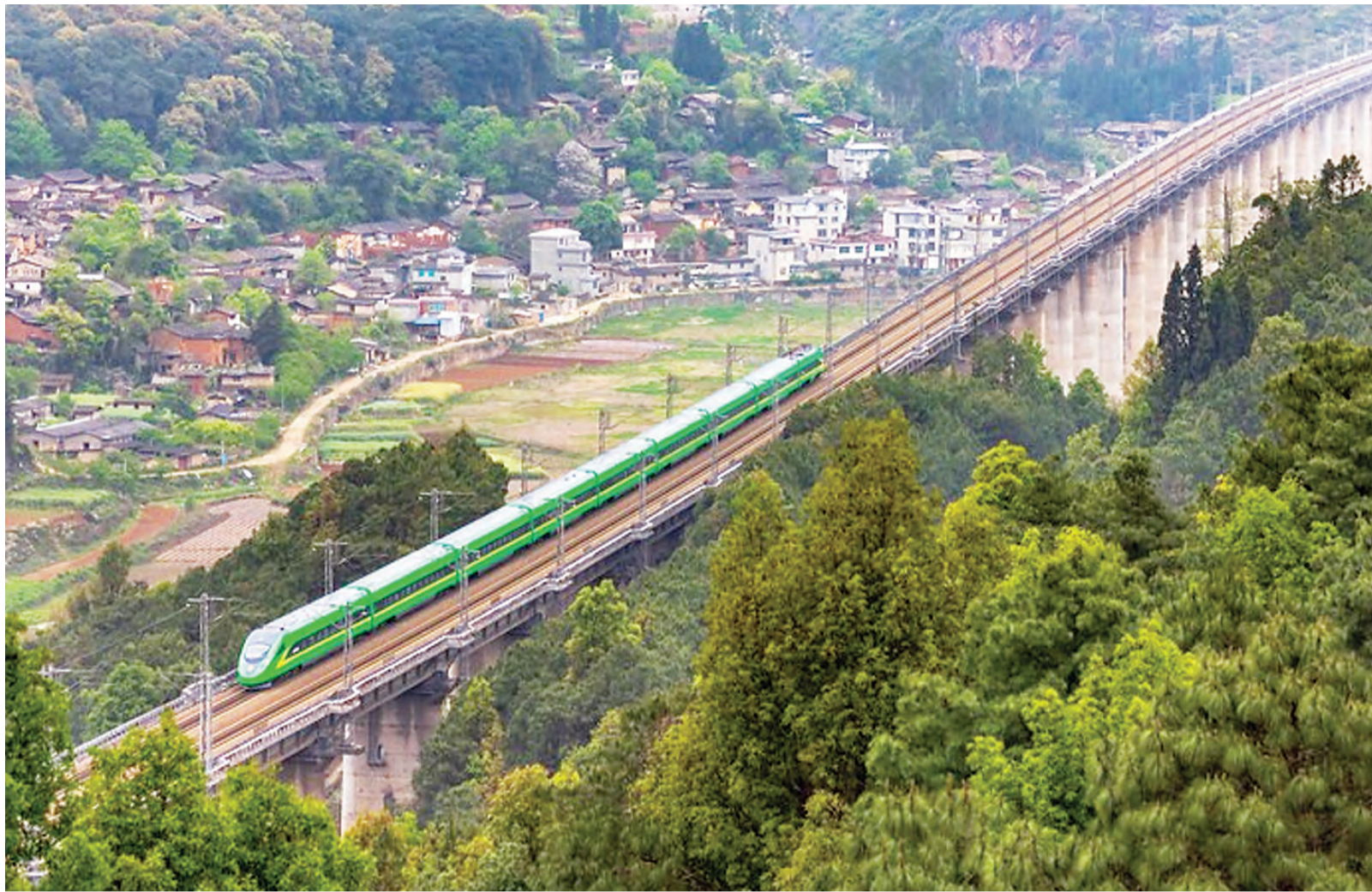
A Fuxing bullet train runs on China's section of the China-Laos Railway on Jan 27, 2023. (PHOTO / XINHUA)
