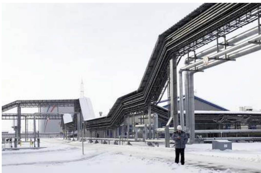
An oil storage tank of Russian oil pipeline monopoly Transneft is pictured at the Baltic Sea port of Ust-Luga, Russia February 26.
