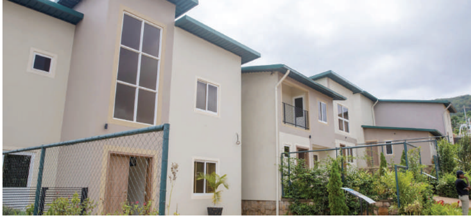
Some of the housing units at Bwiza Riverside Estate in Nyarugenge District
