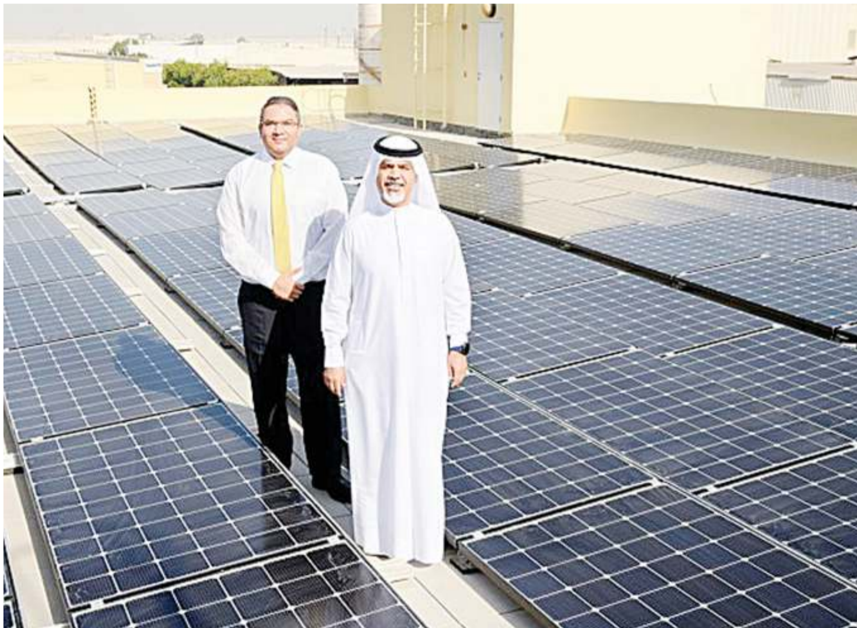
An EKFC state-of-the-art solar power system in Dubai.
