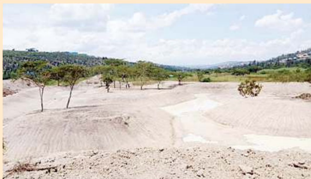
Nyandungu Urban Wetland Eco-Tourism park project is under construction.
