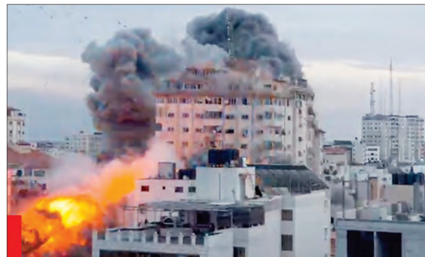
Massive explosion as Gaza high-rises destroyed by jets
