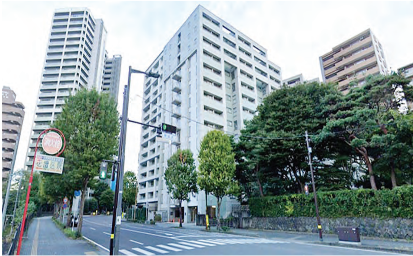
S-Fort Katahira was completed in 2006 and is the newer of AXA IM's two Sendai acquisitions.
