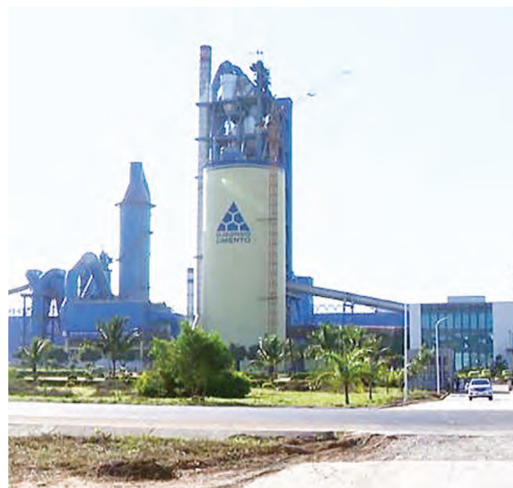
Dugongo Cement Plant in the southernmost district of Matutuine, Mozambique.
