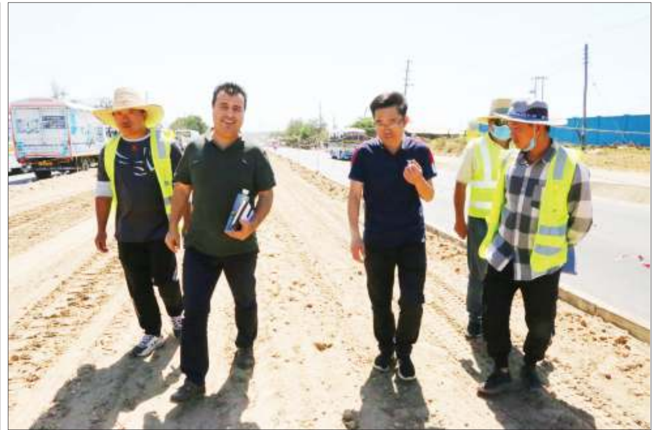
Work on Phase II of the Dar es Salaam Rapid Transport (bus) project began along the city's Kilwa Road at the weekend under China's Sino Hydro firm, whose engineers are pictured engaged in consultations at the Mbagaia Kizuiani site on Monday. Photo: Selemani Mpochi
