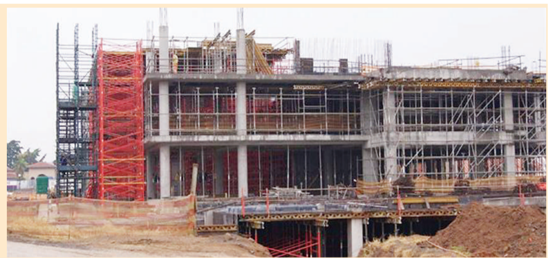
Tlhabane Square development in Rustenburg.
