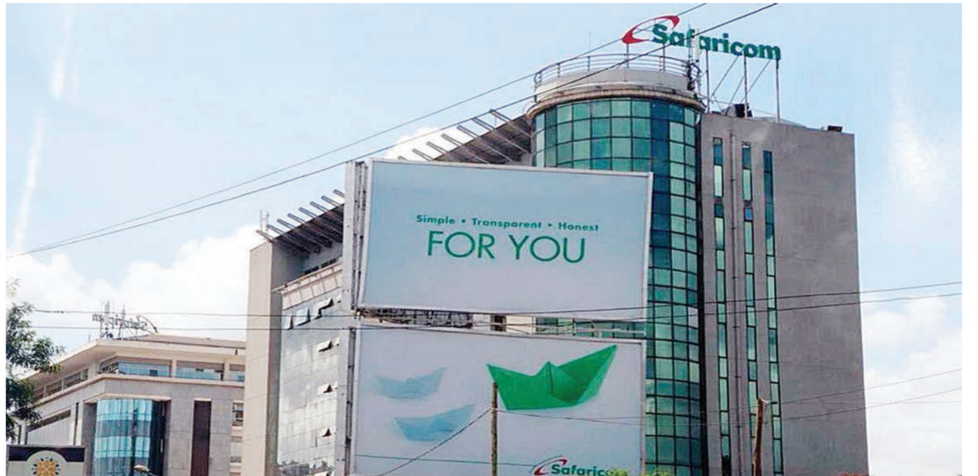
Safaricom PLC headquarters in Westlands, Nairobi.
