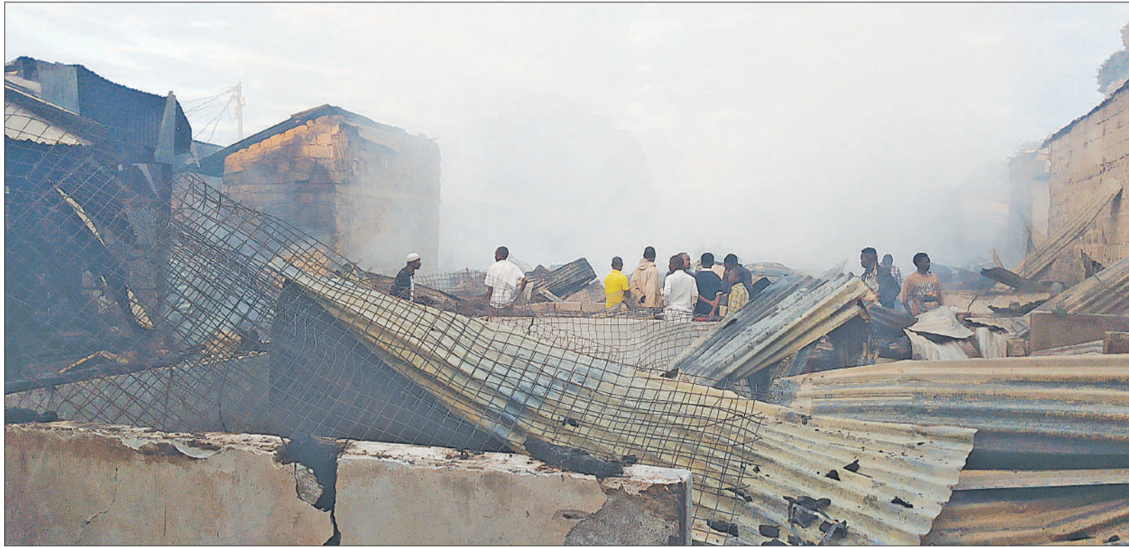
This is the debris of buildings housing at least 100 kiosks at Masasi Town Council's main market gutted by fire on Tuesday night. No details on the incident have been established. Photo: Correspondent Hamisi Nasri
