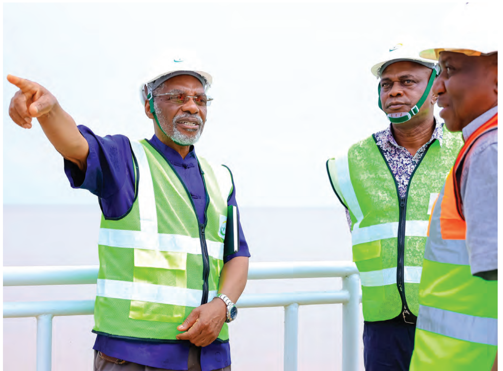
Tanzania Electric Supply Company (Tanesco) Board member Prof Idris Kikula (L) and colleagues pictured during a visit to the Julius Nyerere Hydroelectric Power Station site in Rufiji District yesterday. Photo: Correspondent Joseph Mwendapole
