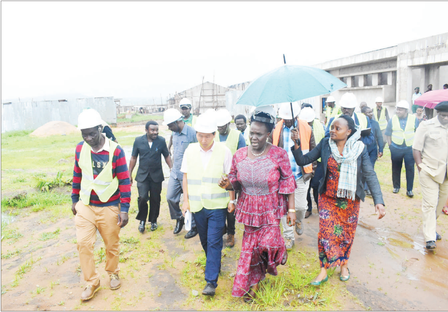
Minister for Education, Science and Technology Prof. Joyce Ndalichako accompanied by civil engineer undertaking the construction of Vocational Education and Training Authority building in Simbawanga district, Rukwa region Ding Fubing (3rd R) during the inspection of the project on Monday. Photo: Guardian Correspondent
