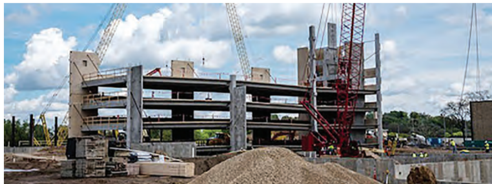
A construction site. File Photo
