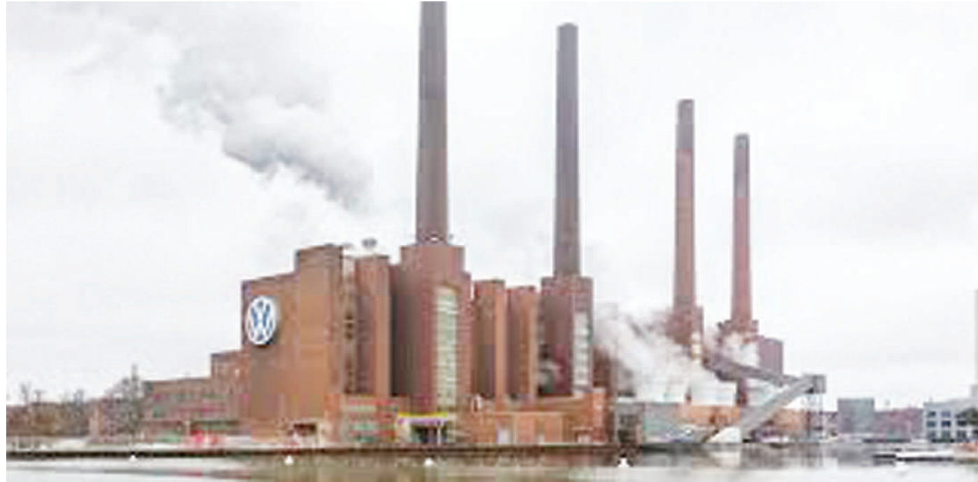
The power station at Volkswagen's Wolfsburg plant in Germany
