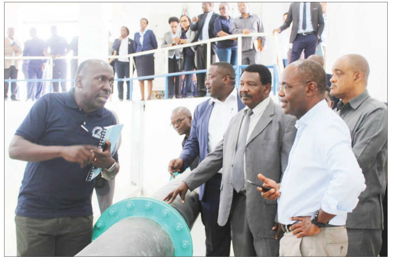
Dar es Salaam Water and Sanitation Authority (Dawasa) engineer Ishmael Kakwezi (L) briefs Water minister Prof Makame Mbarawa (2nd-R, in specs) and the agency's board members on operations at the 10bn/- Dawasa-funded Kibamba-Kisarawe water project at the weekend. Photo: Guardian Correspondent
