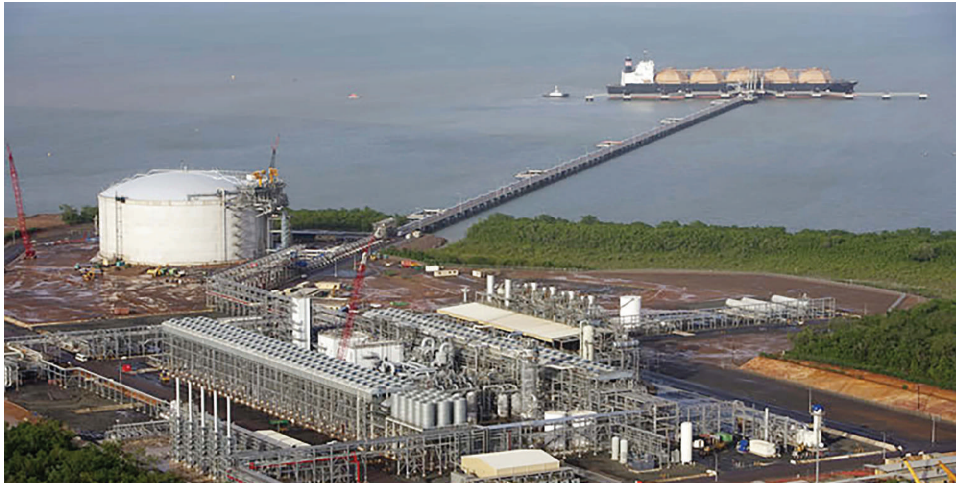
A Liquefied Petroleum Gas offloading facility. Photo: File
