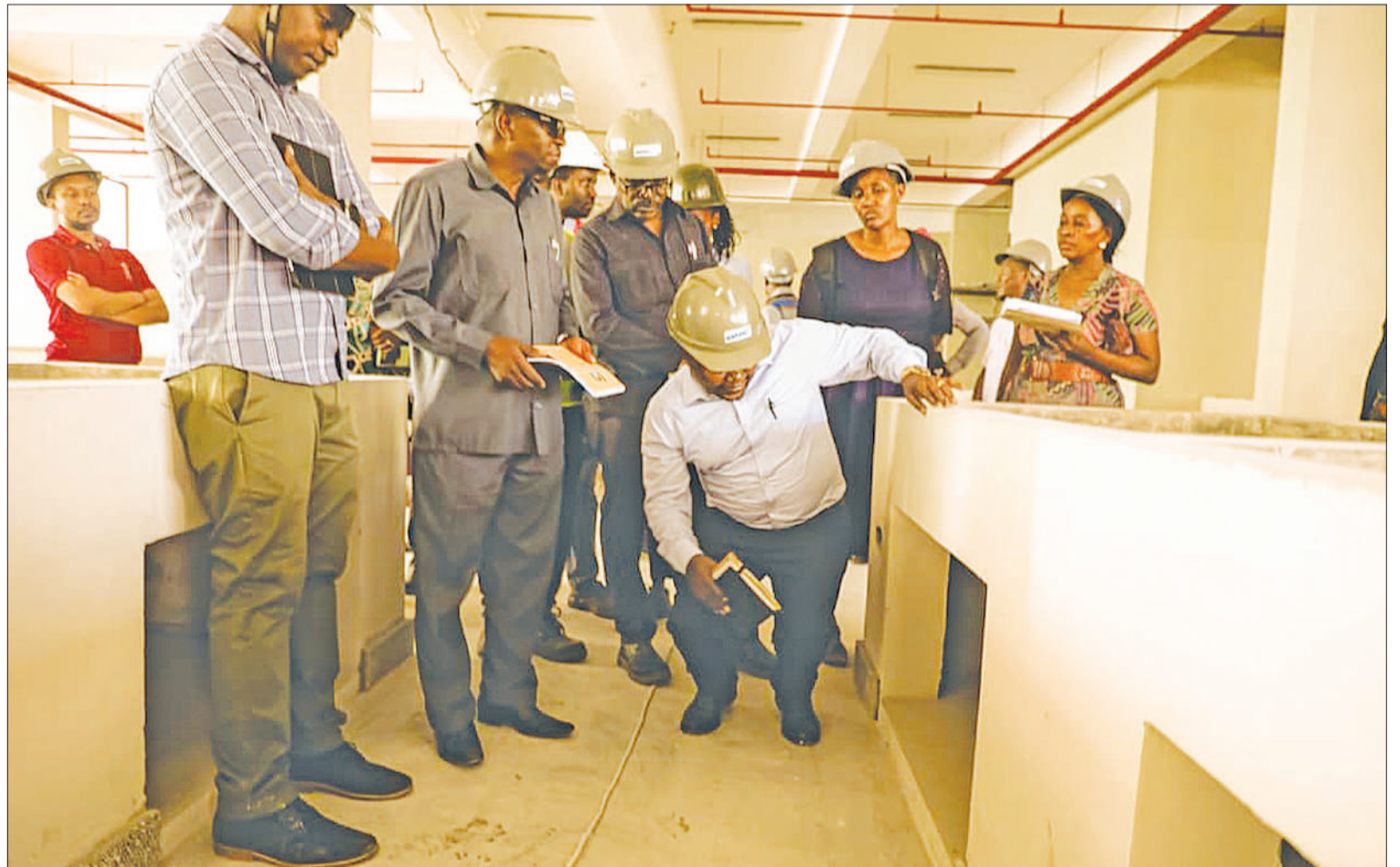
Rogatus Mativila (kneeling), Deputy Permanent Secretary in the President's Office (Regional Administration and Local Governments - Infrastructure), inspects one of the cubicles at Dar es Salaam's mixed-goods Kariakoo market. The complex was gutted by fire, with its rehabilitation now standing at 91 per cent. Photo: Guardian Correspondent
