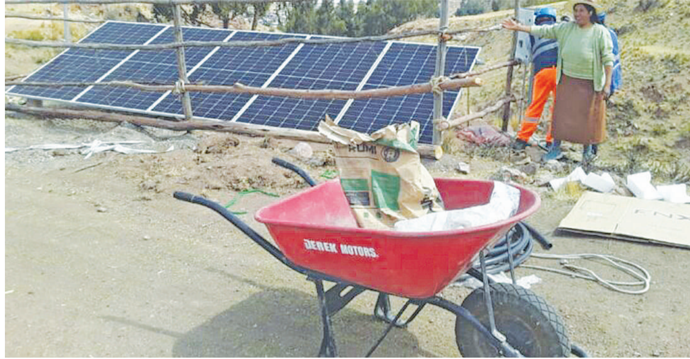
Pumps fueled by 180-watt solar panels draw water from rustic wells to irrigate vegetable crops in the highland greenhouses of Peruvian farming communities. In the picture, farmer Fermina Quispe is helping to move the solar panels. CREDIT: Courtesy of Fermina Quispe
