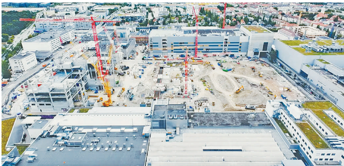
BMW new construction site.
