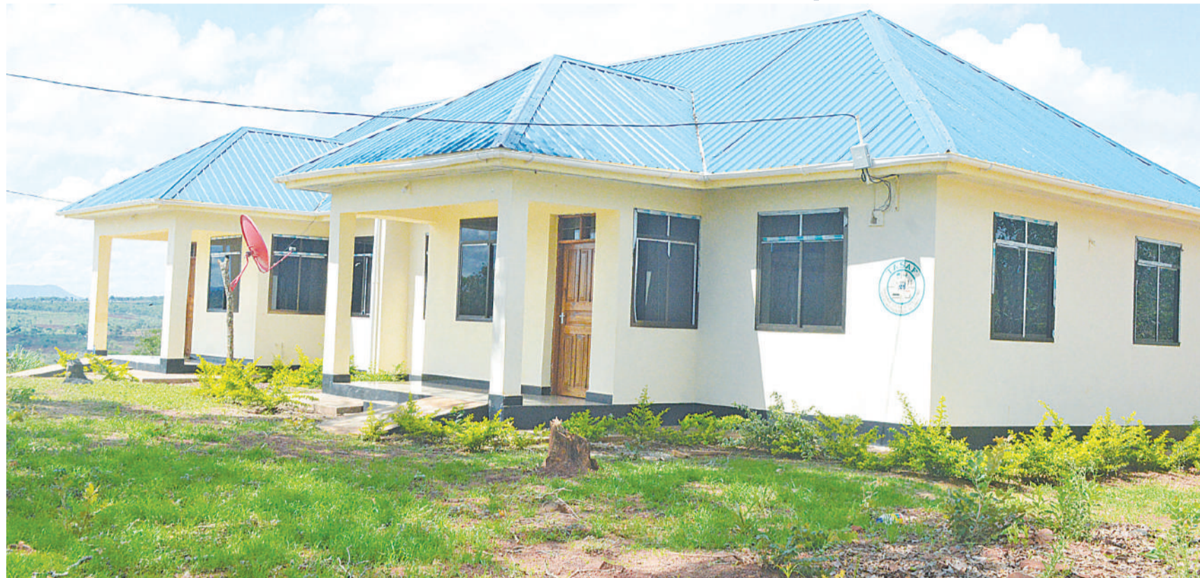
Mdundualo health centre's residential house for nurses and a medical doctor as captured recently in Peramiho District. Photo: Francis Kajubi
