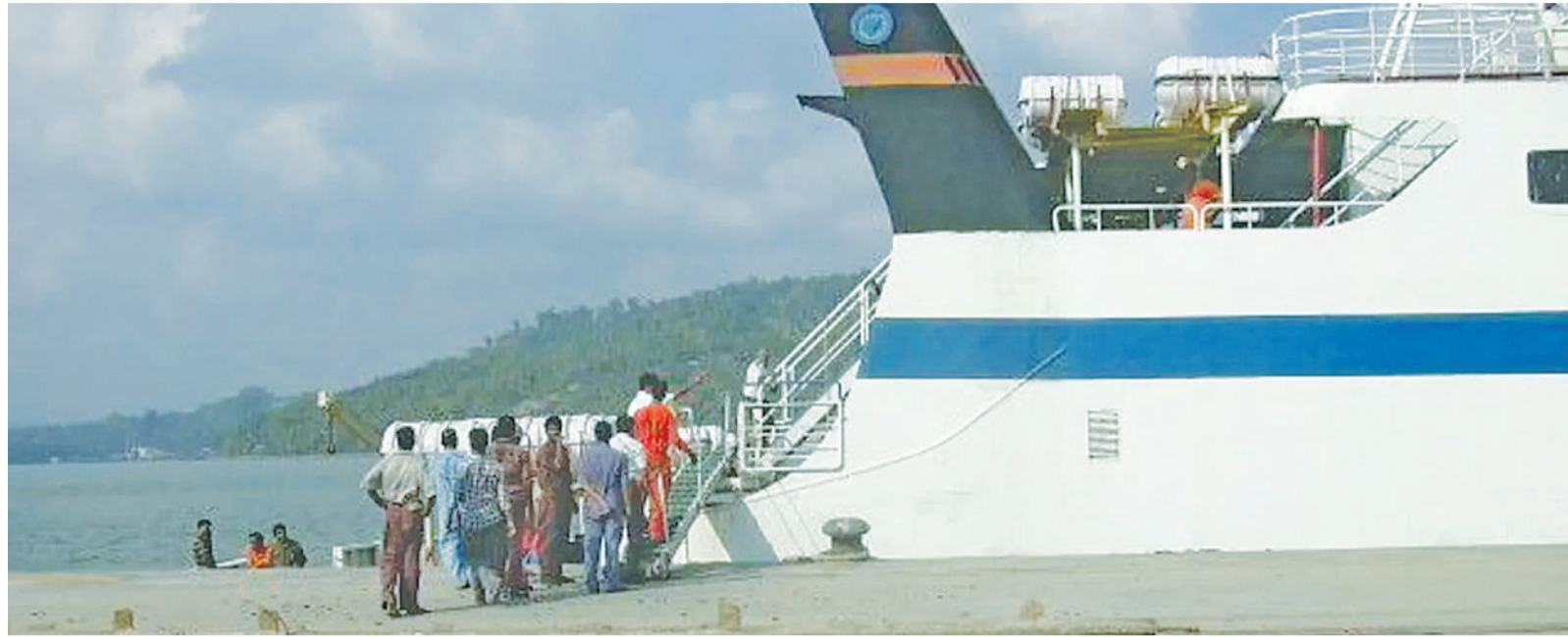
Just as we pulled out from the harbour, our boat lurched and suddenly the jetty next to where we had boarded collapsed into the sea
