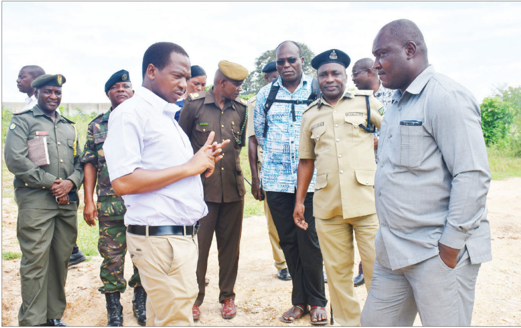
Leopold Runji (L, gesturing), an engineer with the Tanzania Rural and Urban Road Agency, briefs Kinondoni district commissioner Daniel Chongolo (R) in Dar es Salaam yesterday on drainage and other infrastructure at buildings being constructed by the Tanzania Building Agency. Photo: Guardian Correspondent
