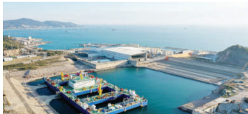
This aerial photo taken on Jan. 30, 2023 shows immersed tube E23 of Shenzhen-Zhongshan highway underwater tunnel and a vessel for its transport and installation at an immersed tube smart factory of CCCC Fourth Harbour Engineering Co., Ltd. on Niutou Island, Zhuhai, south China's Guangdong Province. (Photo by Xinhua)
