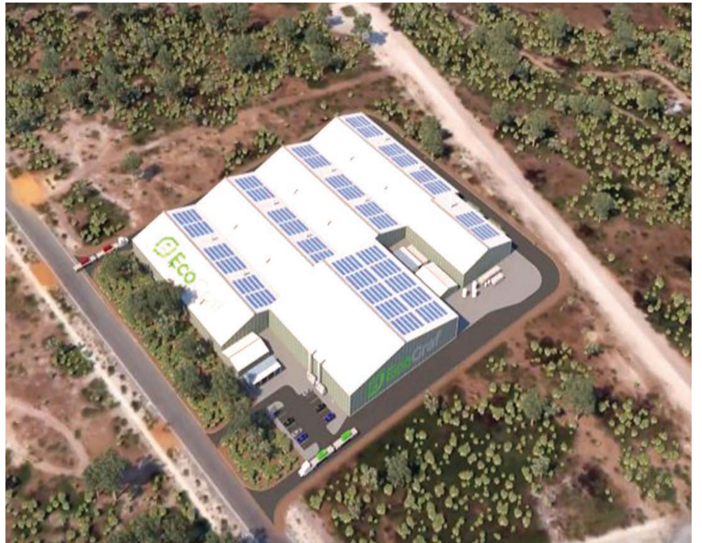
An illustration of EcoGraf's battery graphite manufacturing facility at Kwinana in Australia.
