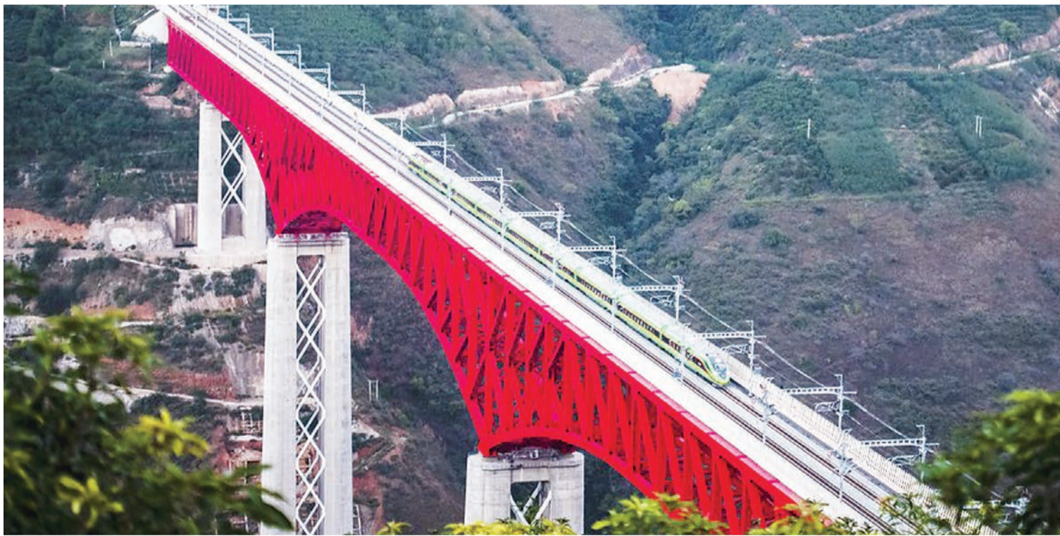
An electric multiple unit (EMU) train of the China-Laos Railway crosses a major bridge over the Yuanjiang River in southwest China's Yunnan Province, Dec. 3, 2021. File photo
