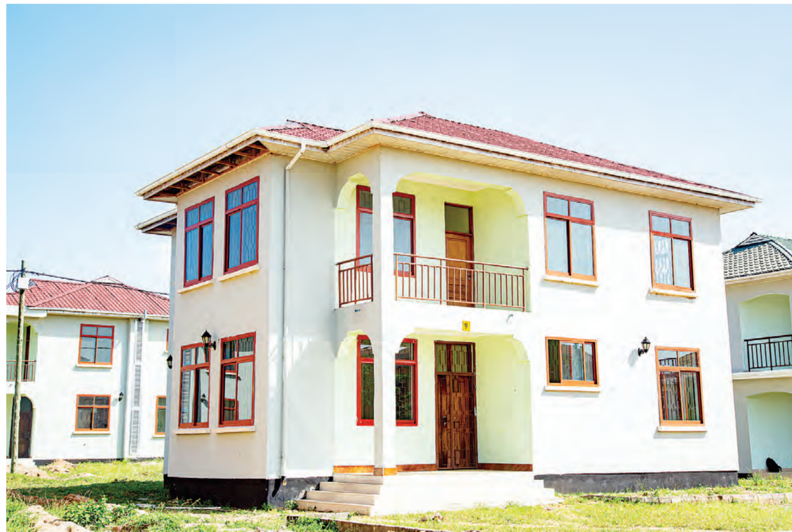
Some of the NSSF houses as part of its investment
