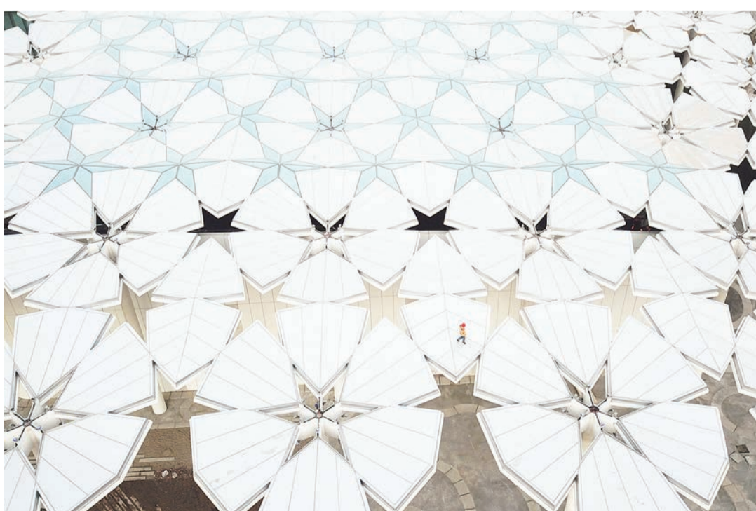
Aerial photo shows a worker walking on the roof of the International Pavilion at the site of the International Horticultural Exhibition 2019 Beijing China (Expo 2019 Beijing). (Xinhua)
