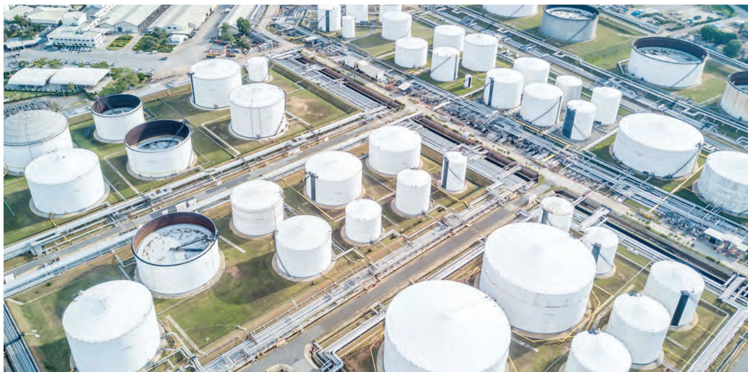
Crude oil storage tanks in China
