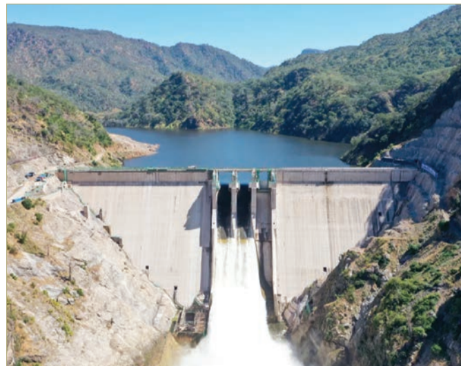
The first unit of the Kafue Gorge Lower Hydroelectric Project in Zambia constructed by the Power Construction Corporation of China is commissioned, June 30, 2021. (Photo by the Power Construction Corporation of China)
