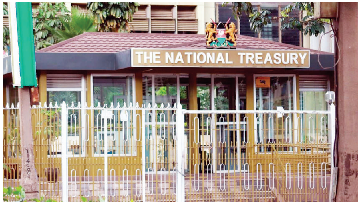
The National Treasury building in Nairobi
