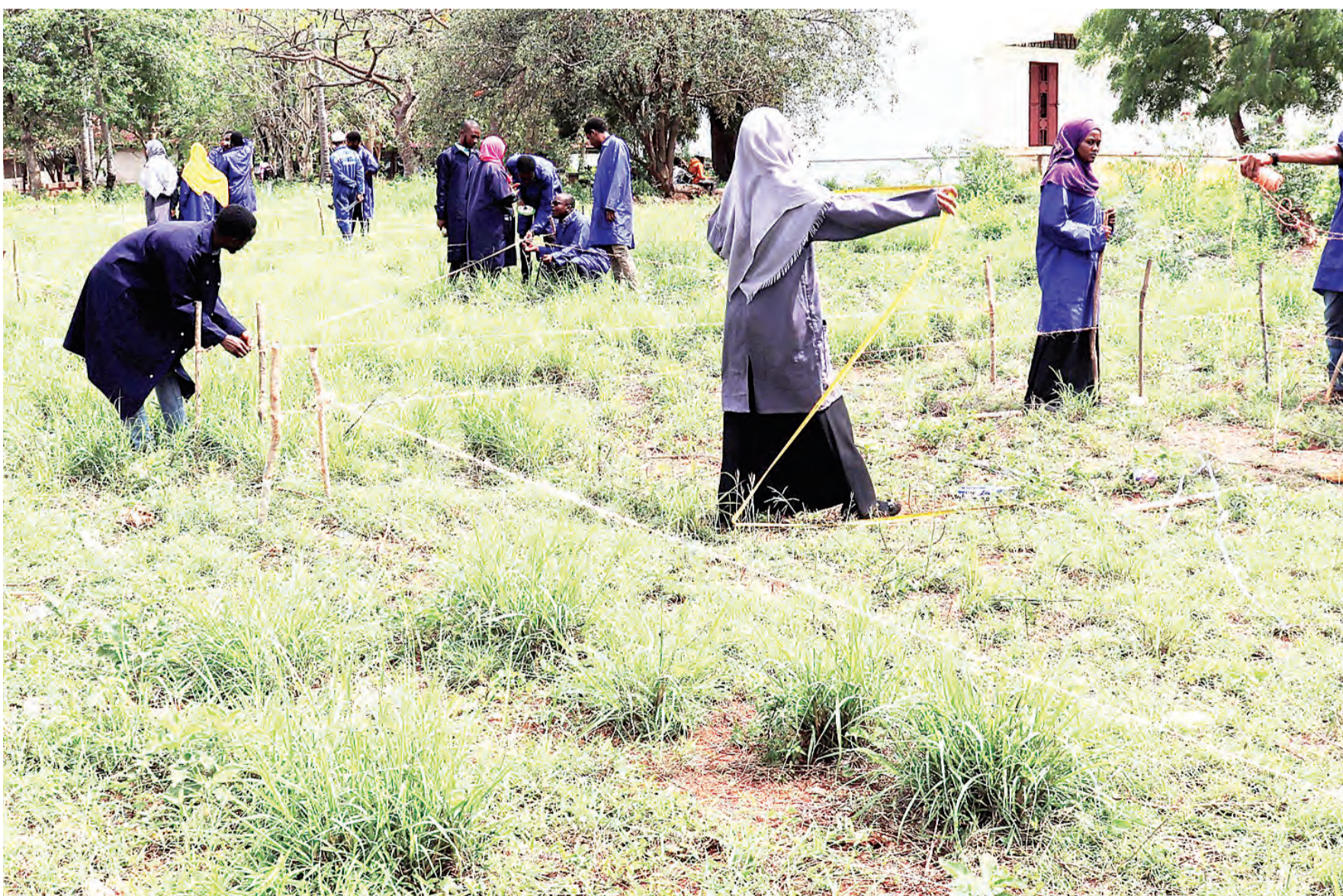
Karume Institute of Science and Technology (KIST) the first year civil engineering degree students on practical training for house construction at Mbweni in Zanzibar yesterday. Photo: Correspondent
