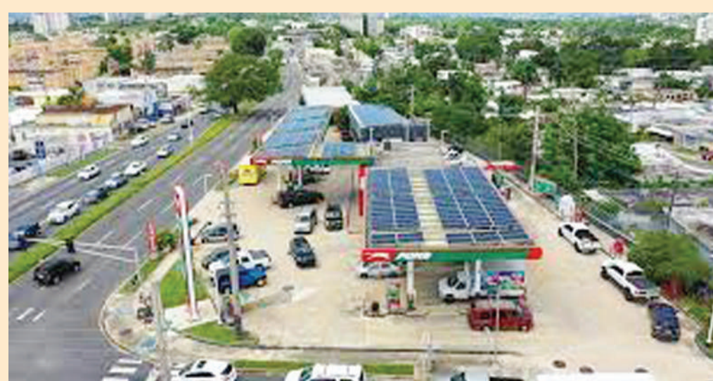
One of the Africa's Puma Energy sites installed solar power panels
