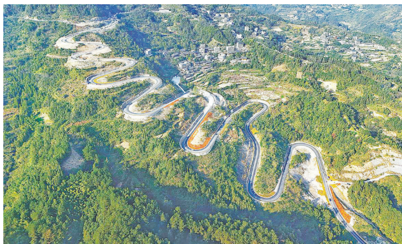
An aerial photo shows a newly built road on Xianglu Mountain in Kaili, a city in southwestern China's Guizhou province.
