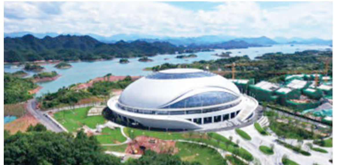
Photo taken on June 14, 2021 shows the track cycling venue of the 19th Asian Games Hangzhou 2022 in Chun'an county, Hangzhou, capital of east China's Zhejiang province.
