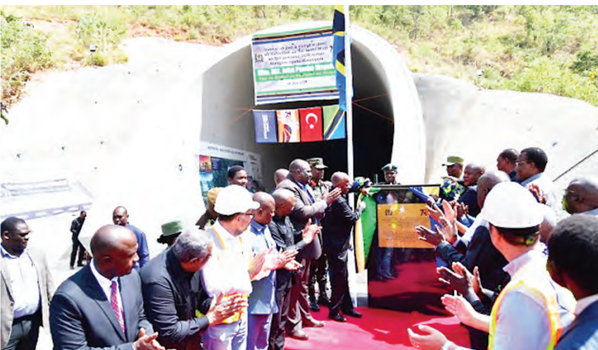
The head of state draws the curtain to launch work on the Standard Gauge Railway tunnel in Kilosa, Morogoro Region.
