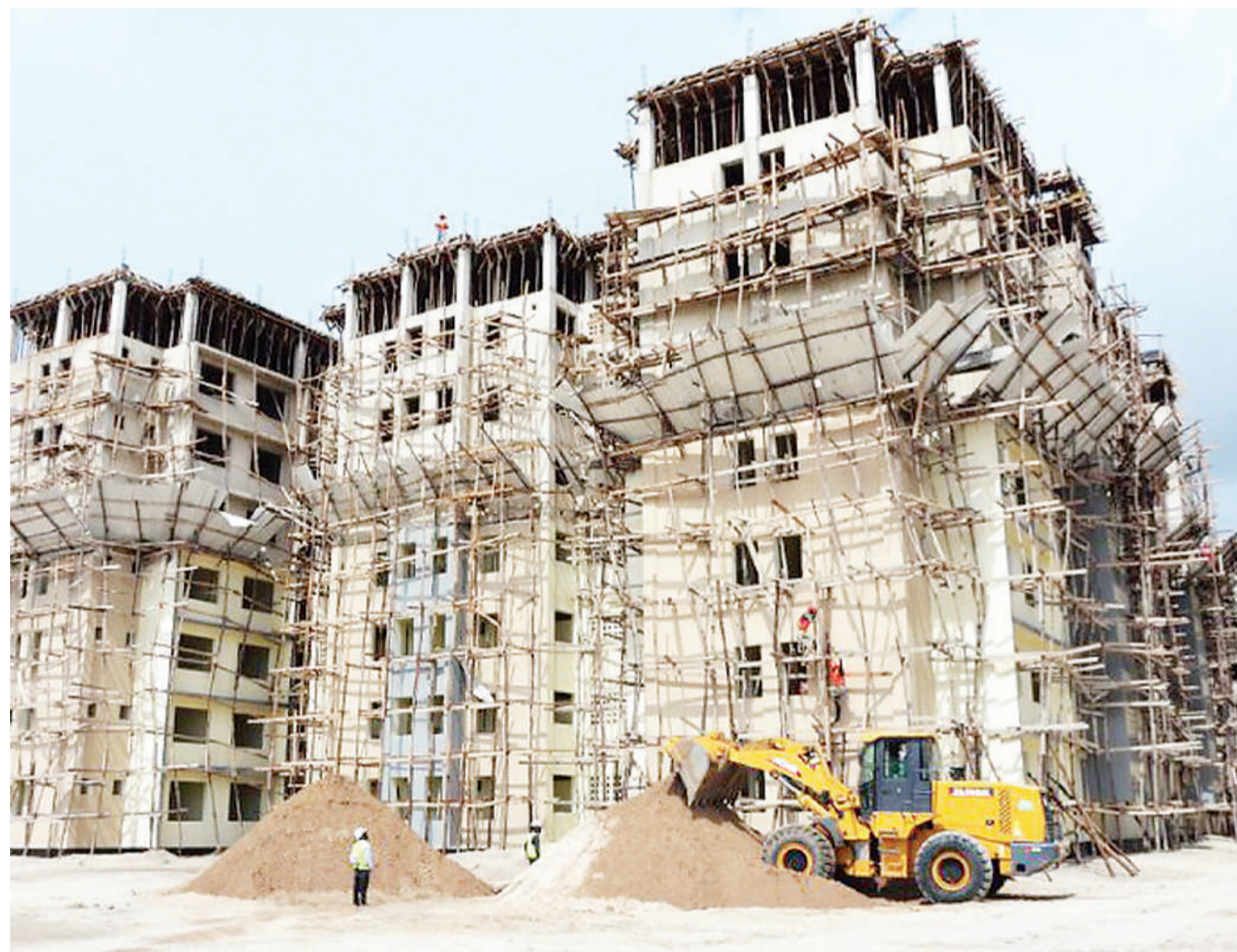
Magomeni Quarters apartments still under construction in Dar es Salaam.
