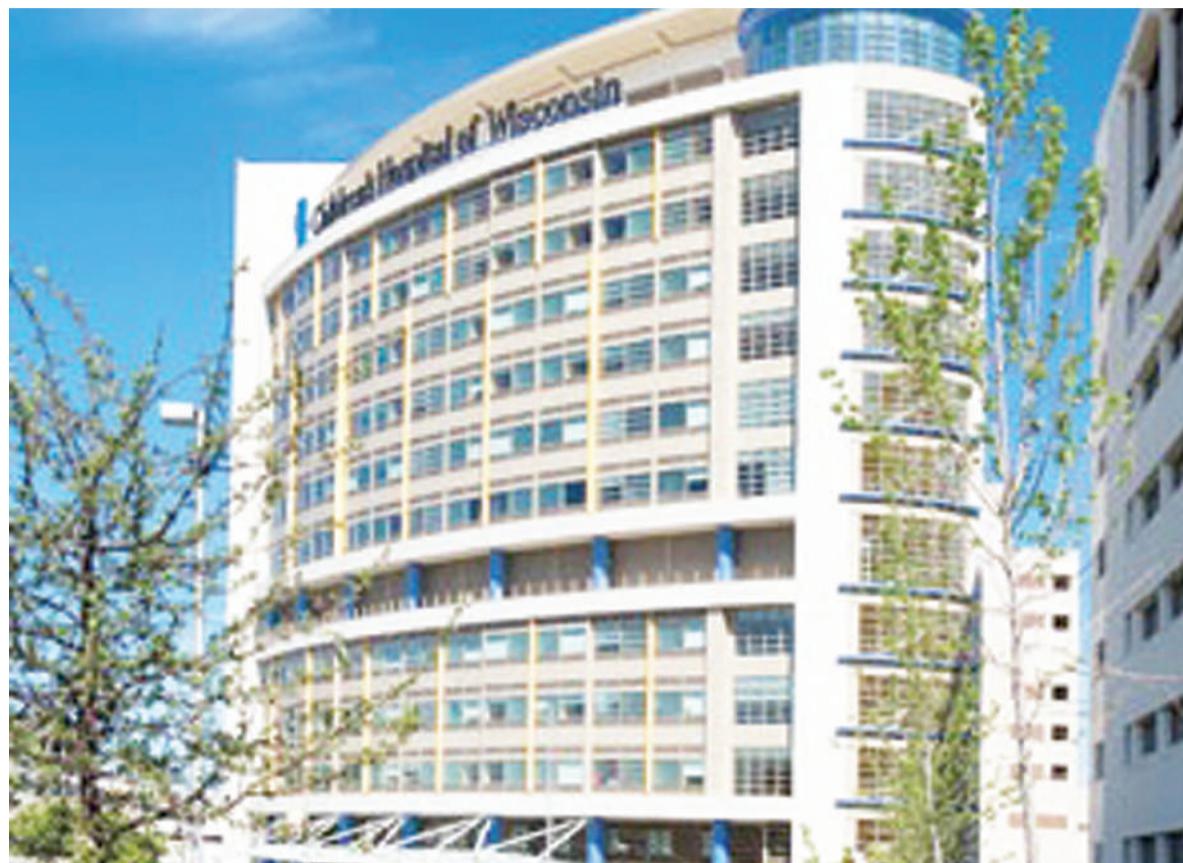
Children's Hospital of Wisconsin, where Boldt used OpenSpace to show construction progress
