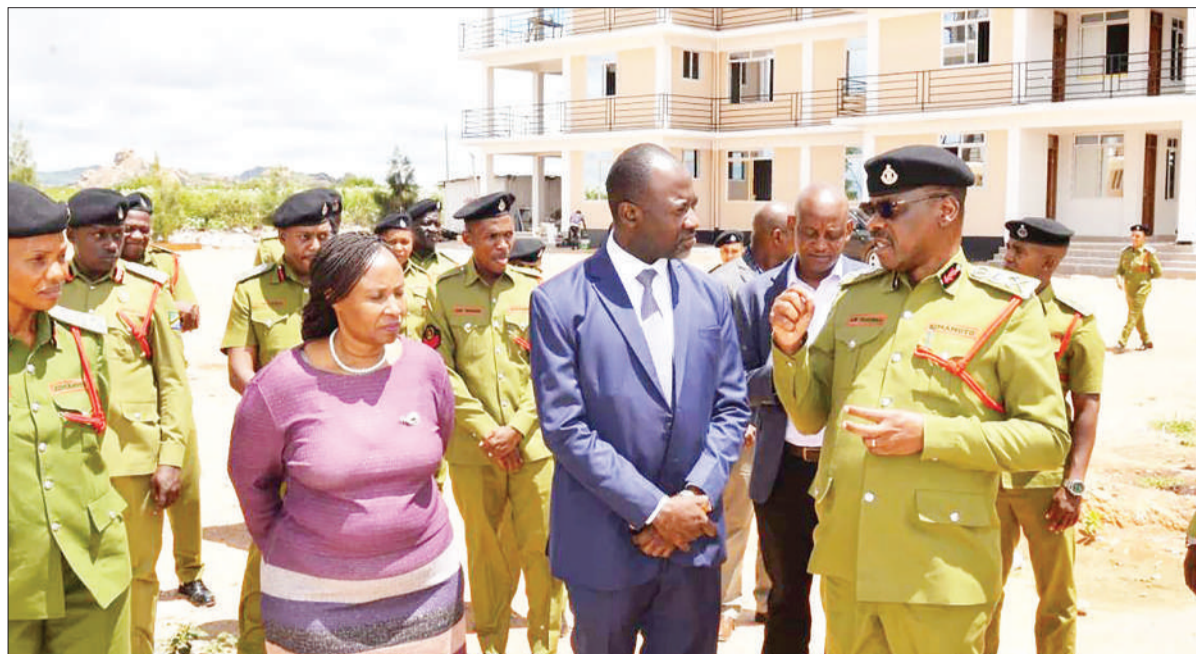
Ally Gugu, (2nd R), the Home Affairs permanent secretary, listens to John Masunga, the Fire and Rescue Force commissioner general, shortly after inspecting the construction project for six storey buildings for staff houses already completed at Kikombo area in Dodoma yesterday. A total of 60 families will be housed in the staff quarters. Photo: Courtesy of the Ministry of Home Affairs
