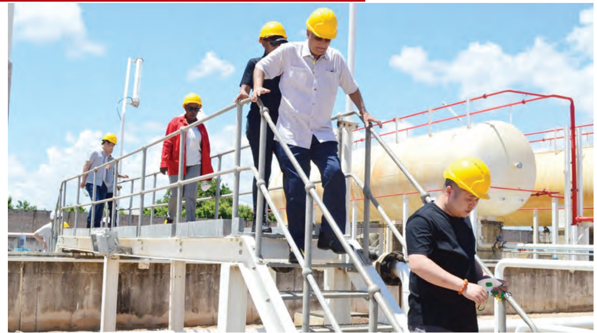
Participants at the two day international gas forum in Dar es Salaam viewing Oryx Gas installations at Kigamboni part of exchanges on the gas sector over the weekend. Photo: Guardian Correspondent
