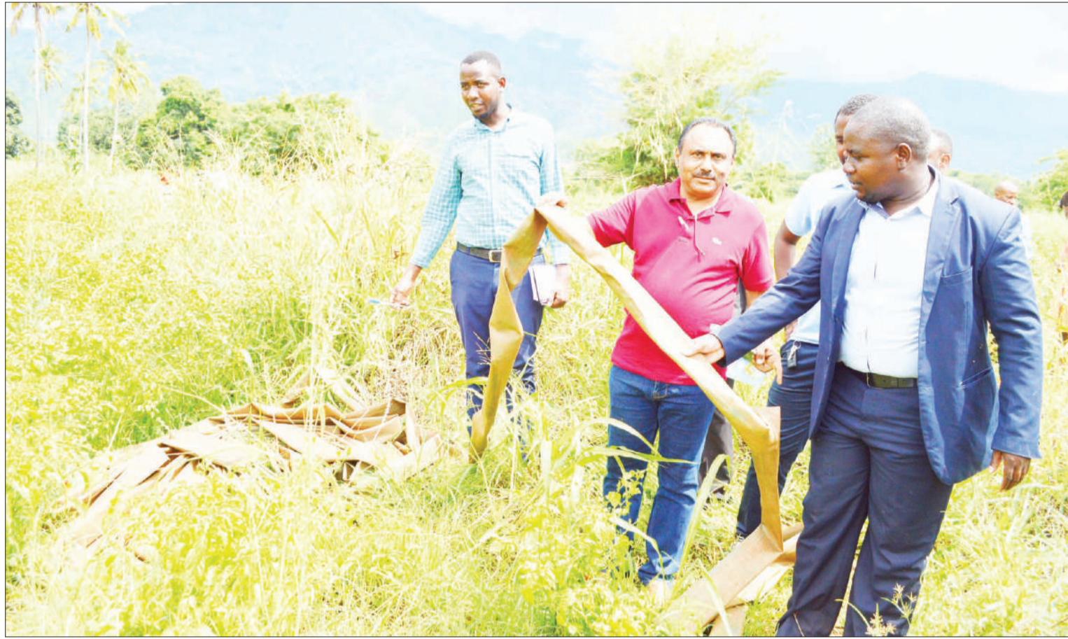
Morogoro Water Supply and Sanitation Authority managing director Tamim Katakwebwa (R) briefs Morogoro Urban legislator Abdulaziz Abood (2nd-L) at the weekend on a water pipe used by farmers to draw water from Mindu Dam for the irrigation of their farms inside 500 meters contrary to the law governing water sources. Photo: Correspondent Ashton Balaigwa
