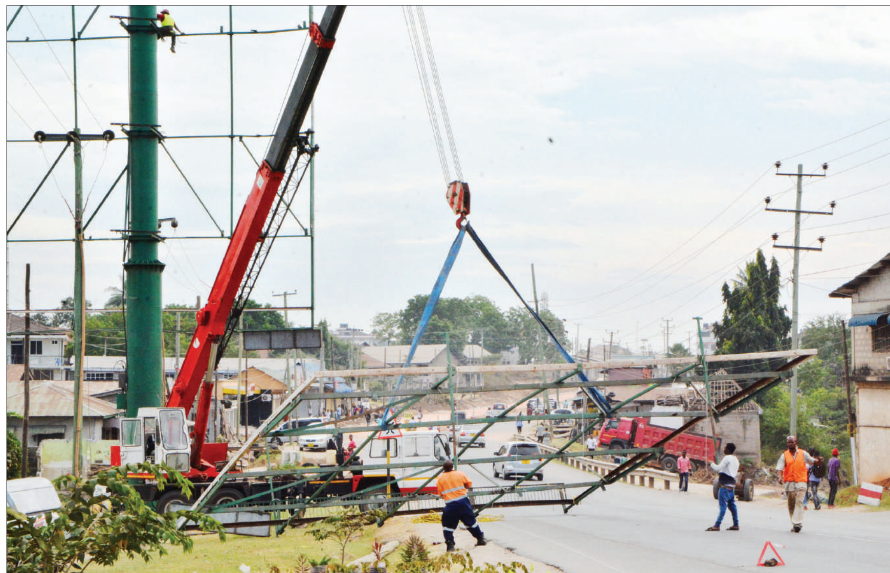
Outdoor billboards are pulled down - pending relocation - to pave the way for the rehabilitation and expansion of the Sinza stretch of Dar es Salaam's Shekilongo Road, as found yesterday. Photo: Correspondent Miraji Msala
