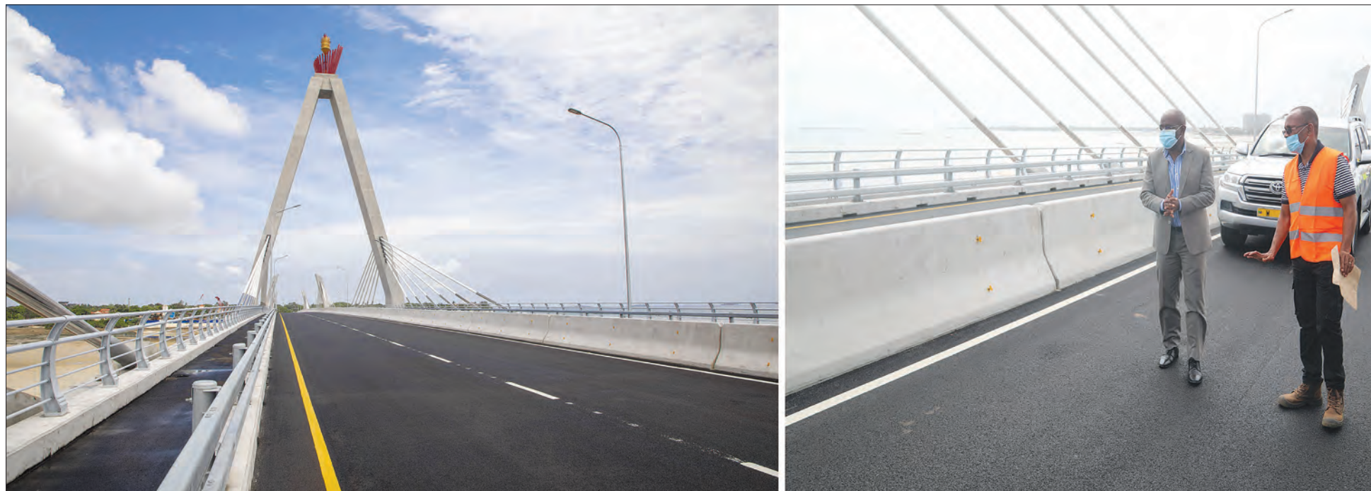
Works and Transport minister Prof Makame Mbarawa (L) pictured yesterday making a confirmatory inspection tour of Dar es Salaam's newly built 2.63-km 256bn/- Tanzanite Bridge. The bridge, built thanks to joint funding by the Tanzanian and South Korean governments, is set to come into use officially beginning tomorrow - as scheduled. It is widely expected ease traffic congestion appreciably, particularly along Ali Hassan Mwinyi Road and Barack Obama Road. He is with Tanzania National Roads Agency (Tanroads) CEO Rogatus Hussein Mativila. Combophoto courtesy of Works & Transport ministry
