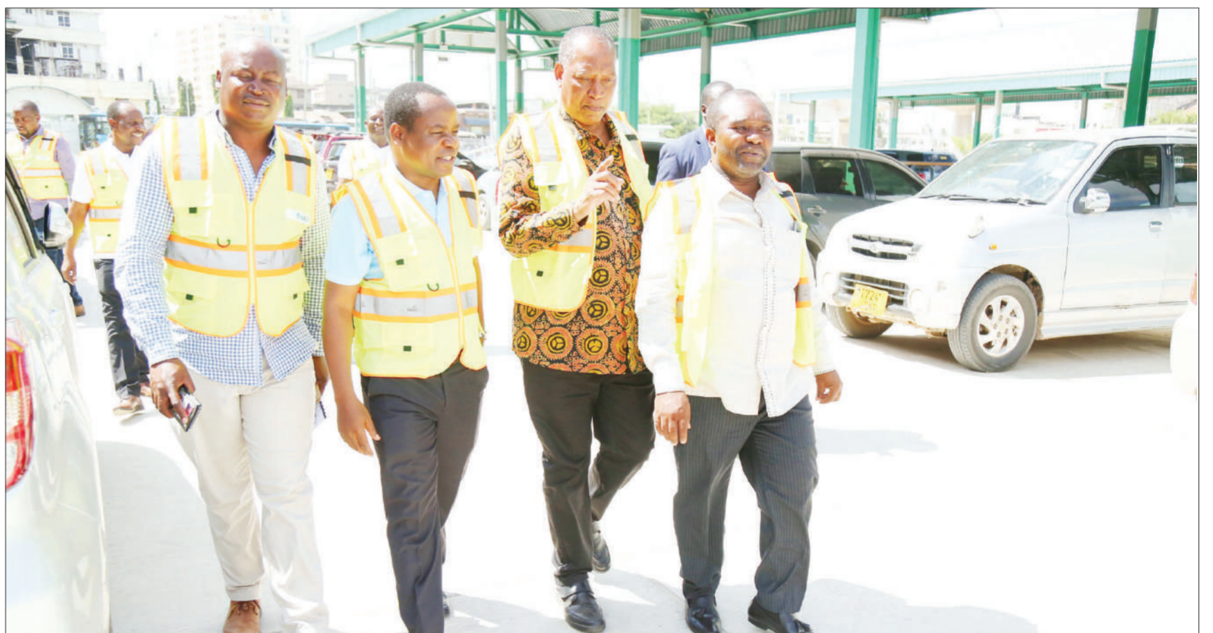
Dar es Salaam Rapid Transit agency (DART) CEO Dr Edwin Mhede (2nd-L) leads members of the Parliamentary Administration and Local Government Committee, including former minister Prof Palamagamba Kabudi (2nd-R) on an inspection tour of the ongoing construction of the main rapid bus station at Mbagala Rangitatu in Dar es Salaam yesterday. Photo: Correspondent Joseph Mwendapole
